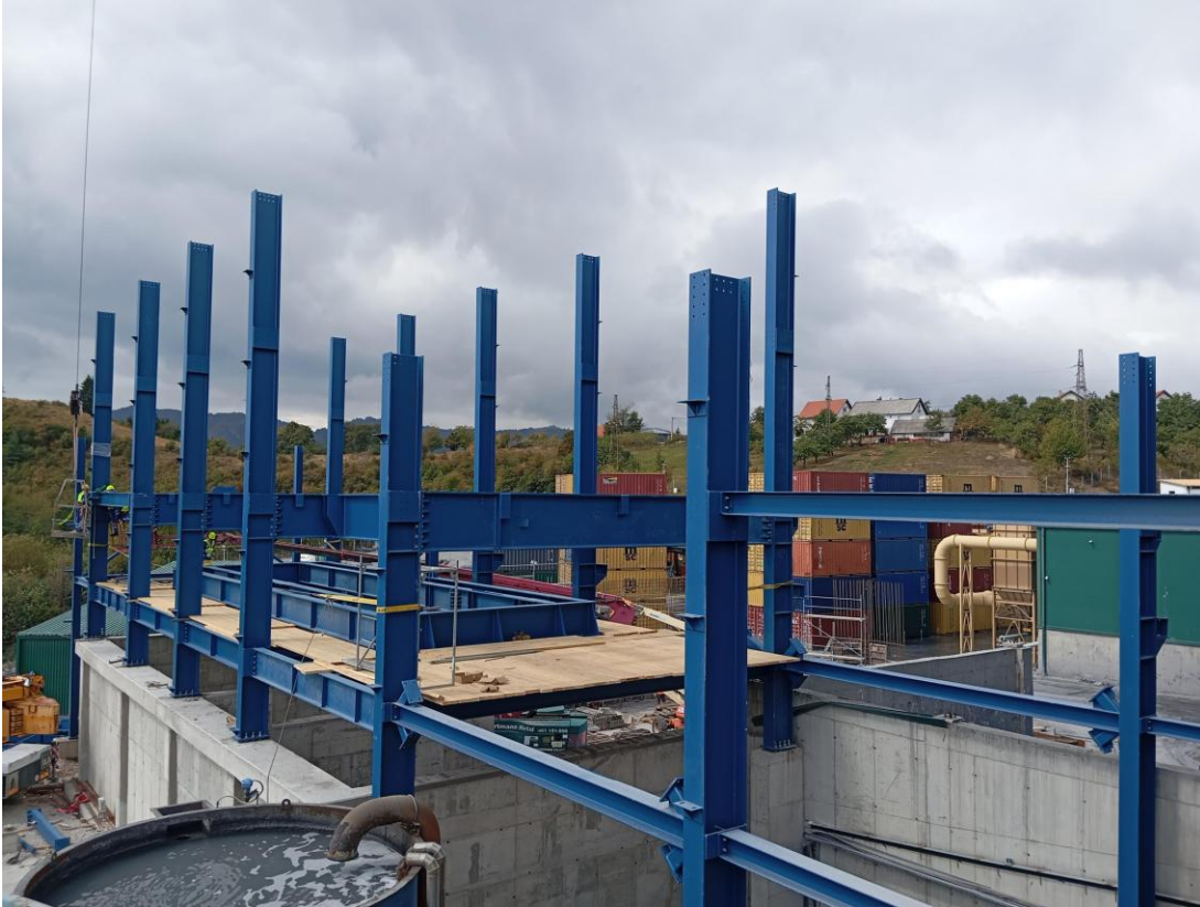
Installation of the second filter press advancing well
