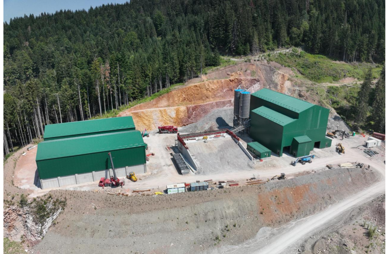
Paste backfill plant nearing completion
