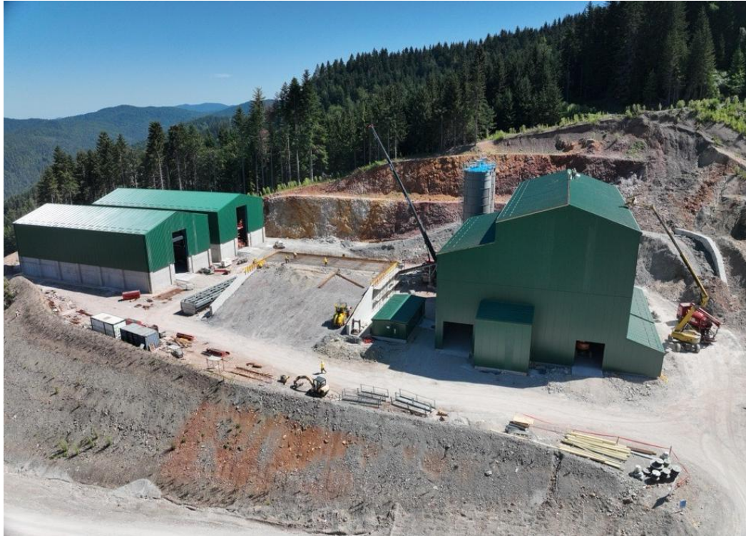
Construction of paste backfill plant advancing well
