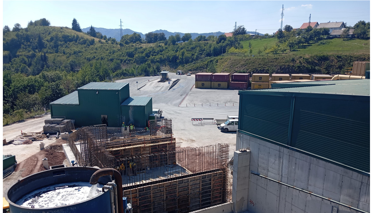
Progressing installation of the second tailings filter press
