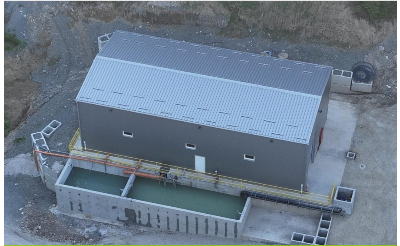
Installation of the water treatment plant
