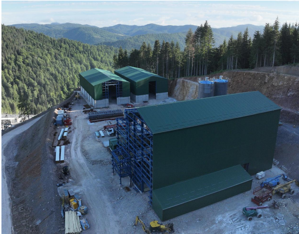
Construction of paste backfill plant advancing well
