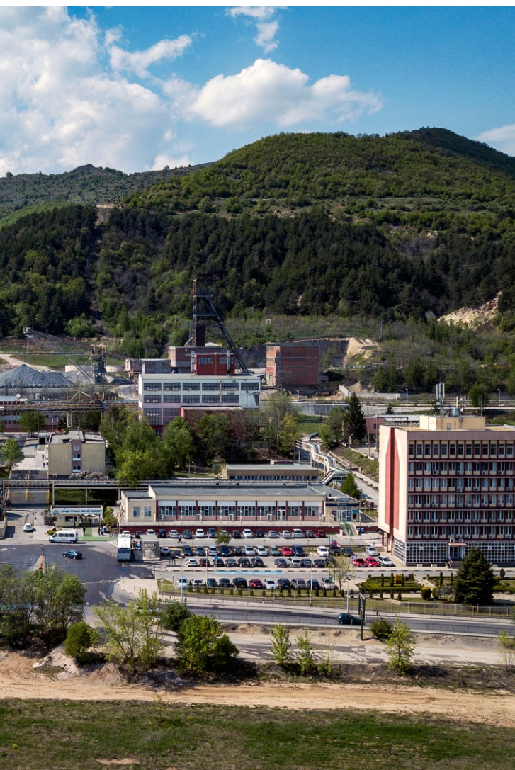
Surface facilities at the Chelopech mine site
