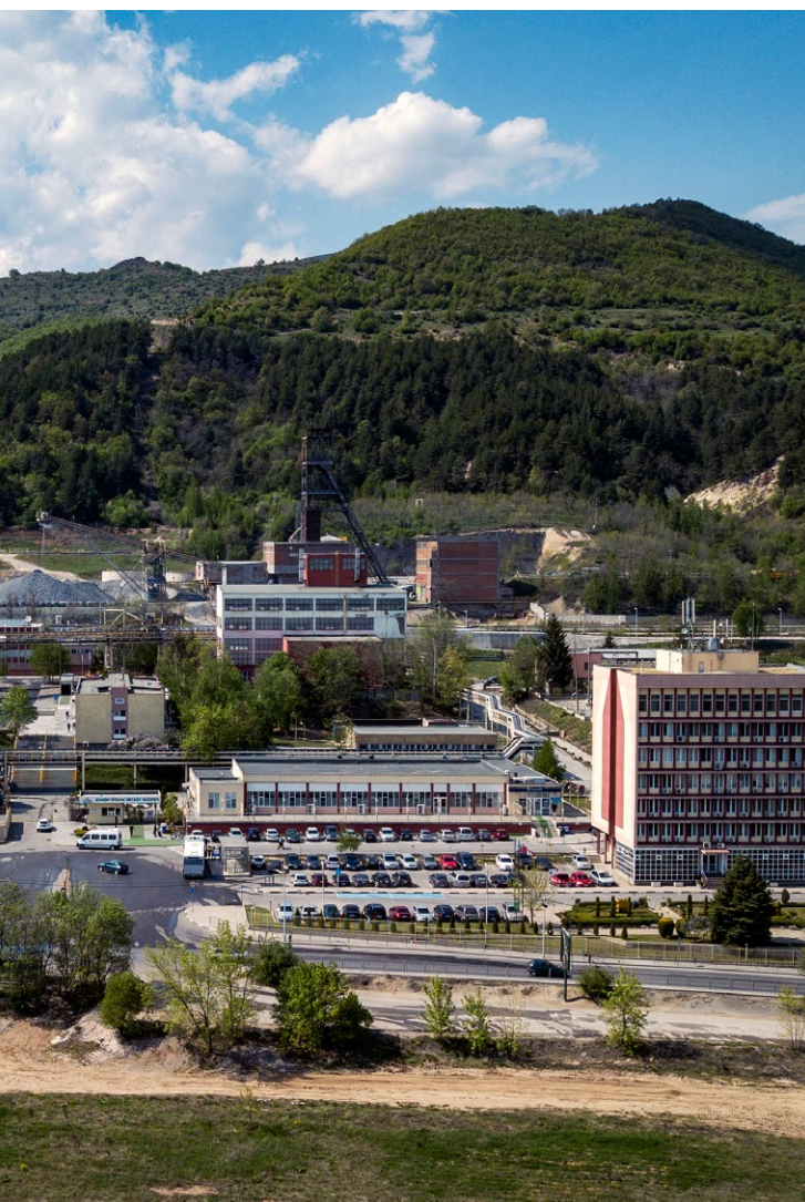
Surface facilities at the Chelopech mine site
