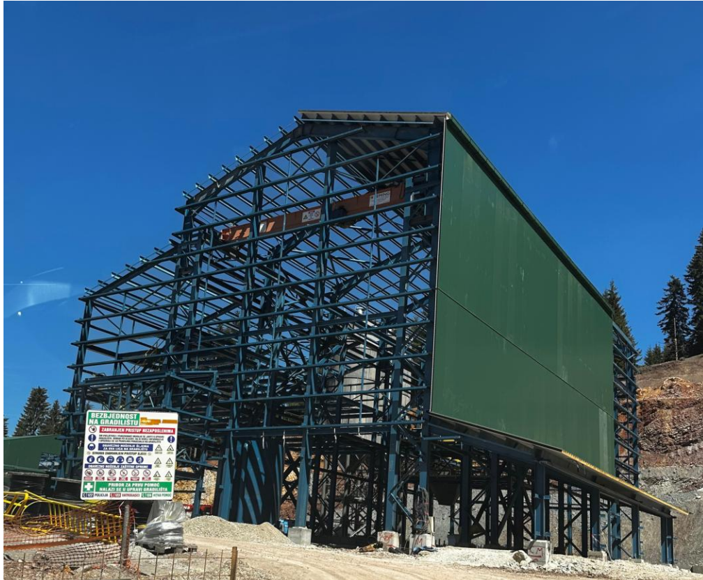
Construction of paste backfill plant advancing well
