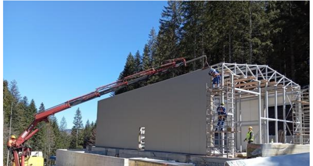
Installation of the water treatment plant
