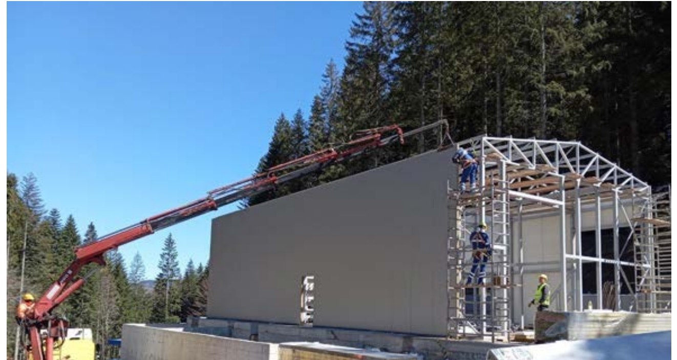
Installation of the water treatment plant
