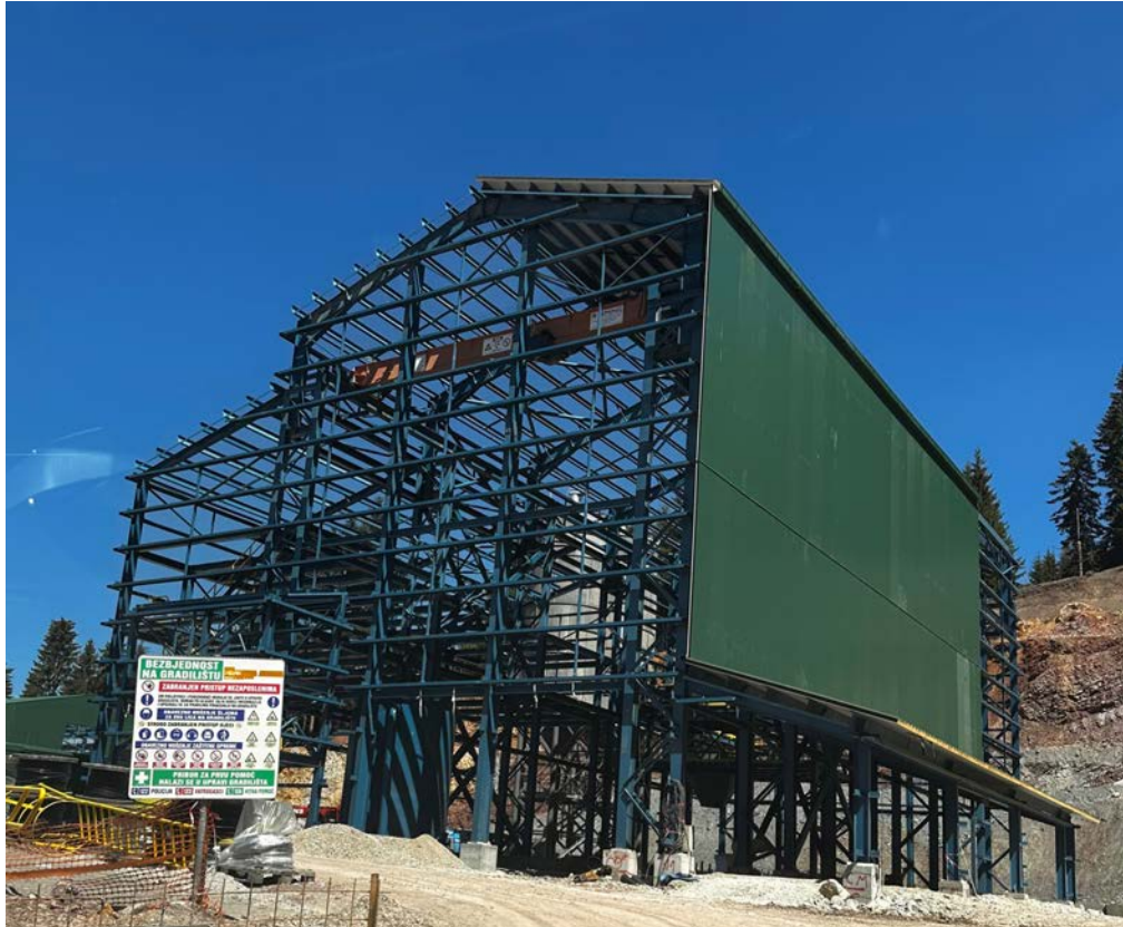
Construction of paste backfill plant advancing well
