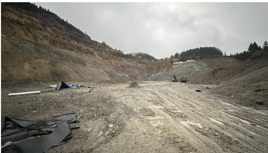
Figure 18-20: Photograph of the Veovaca TSF showing a general view of the TSF development area including the steeply inclined mine void side slopes that will require lining in Phase 1 and Phase 2 (SRK photograph, 25 March 2025, looking north)
