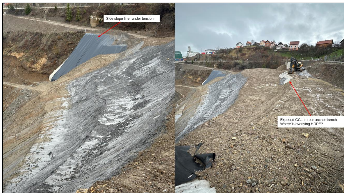
Figure 18-5: Annotated photographs of the Temporary TSF showing condition at the crest of the facility (SRK photograph, 25 March 2025)
