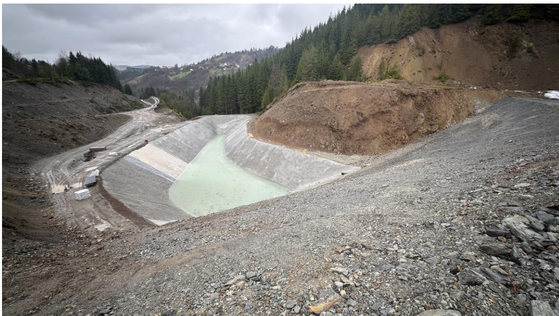
Figure 18-19: Photograph showing a general view of the TSF contact water management pond downstream of the starter dam (SRK photograph, 25 March 2025, looking south)
