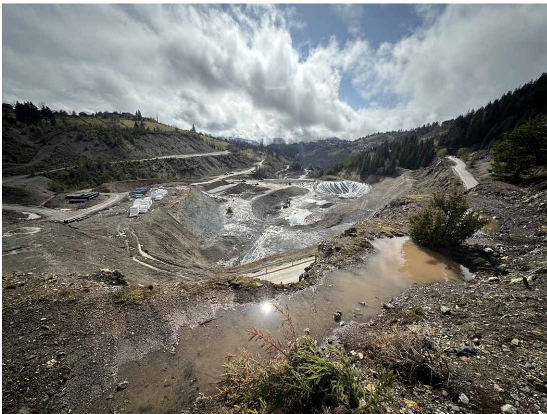
Figure 18-15: Photograph of the Veovaca TSF showing a general view of the TSF development area including the lined topographic bowl behind the starter dam (SRK photograph, 25 March 2025, looking south)
