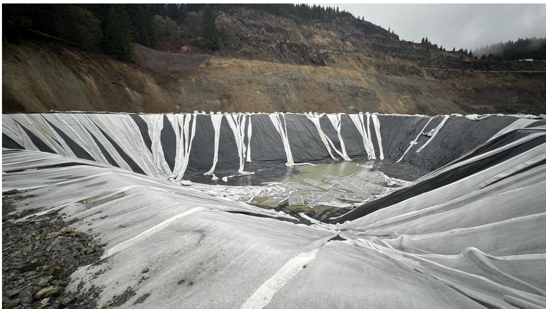
Figure 18-16: Photograph of the Veovaca TSF showing the lined topographic bowl behind the starter dam. While material is the over-liner drainage geocomposite (SRK photograph, 25 March 2025, looking north)
