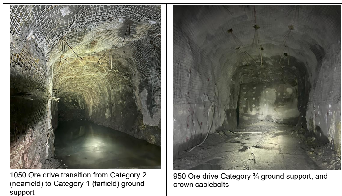
Figure 16-8: Various ground support categories installed (Photographs by SRK)
