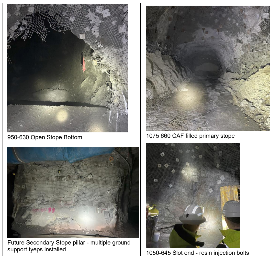
Figure 16-6: Examples of stoping and ground support – 950-1075 levels
