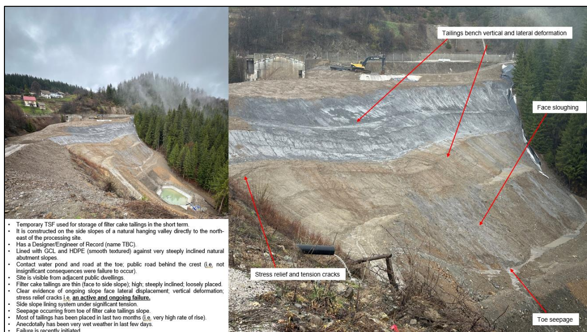
Figure 18-4: Annotated photographs of the Temporary TSF showing location and extent of active slope instability failure (SRK photograph, 25 March 2025)
