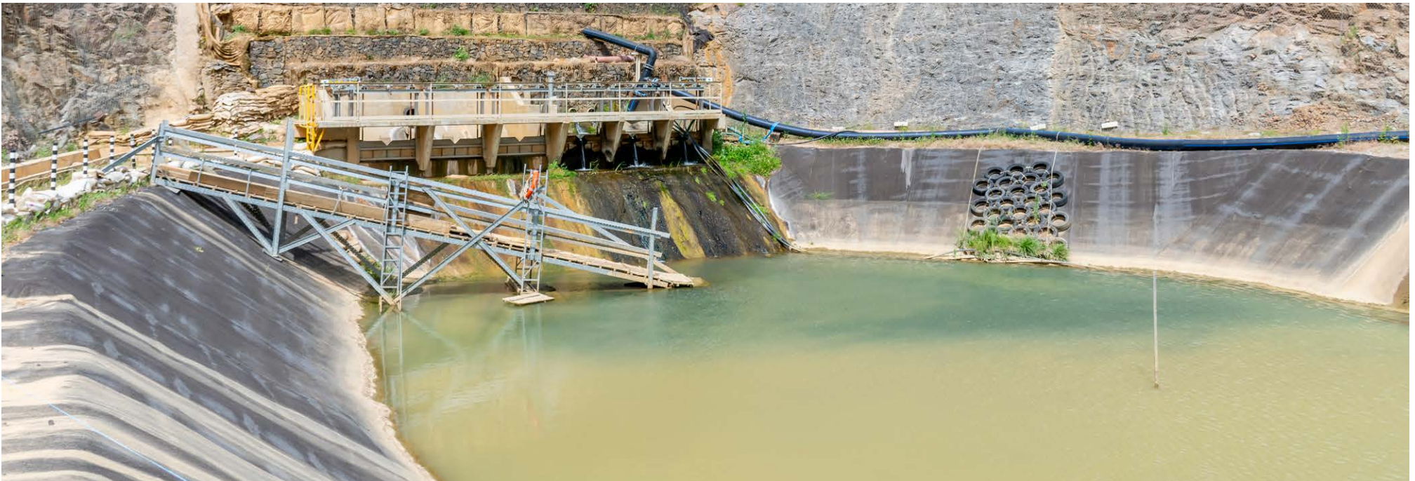
Storm water reservoir overflow at Ada Tepe mine in Bulgaria
